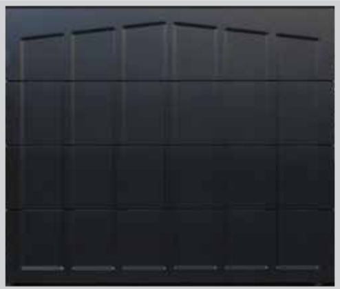
Okoume plywood cladding milled to recreate the specific door design according to conservation area regulations.
